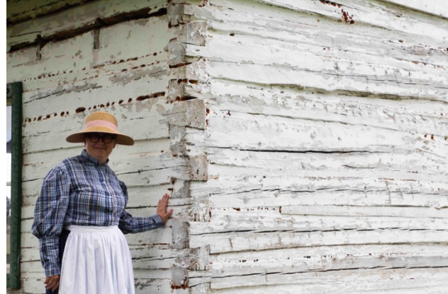
Figure 27. The home in this photo was made using hewn logs, but many traditional houses were made with rounded logs.
